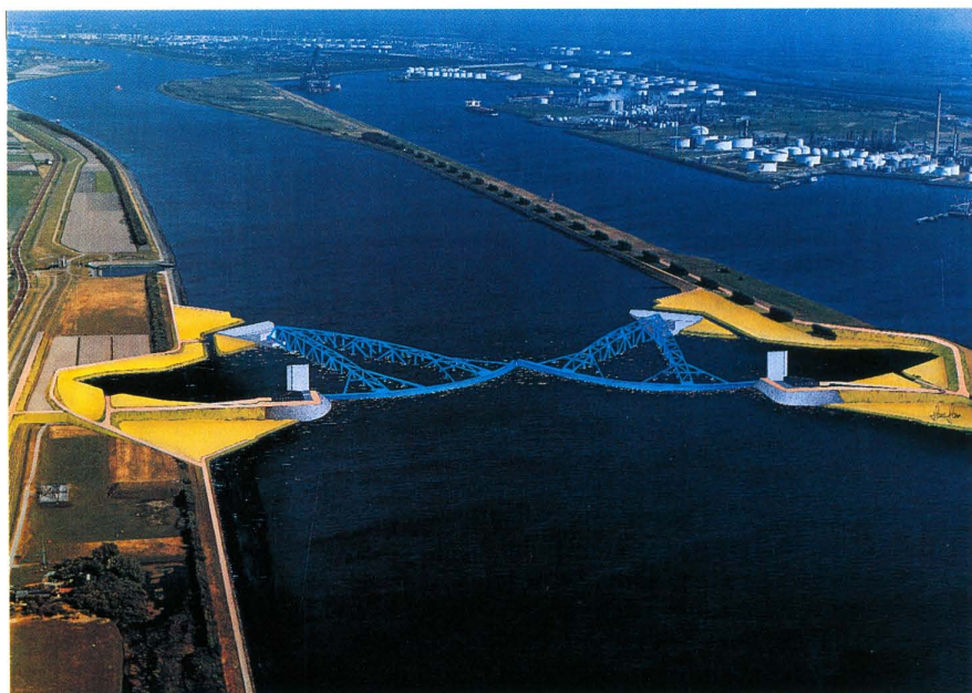
Figure 2. Artist's view of the very large storm surge barrier now under construction in the New Waterway to Rotterdam harbor, one of the world's largest. Closing time for the barrier will be three hours, shutting down traffic for a minimum of six hours. The precision and timeliness of the storm forecasting system will have a direct economic impact.
